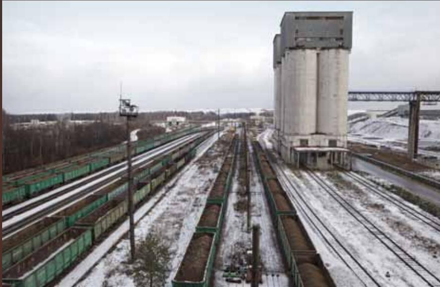
An average of 9 to 13 million tonnes of oil shale annually, that is, an average of 300 to 400 rail car loads daily, are transported to the power plants in Narva. All together, the power plant receives enough oil shale to fill a train 3,500 kilometres long, equal to the travel distance from Tallinn to Barcelona.
