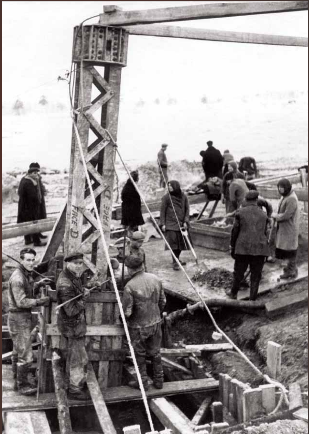
Construction of the station began in the autumn of 1936.
