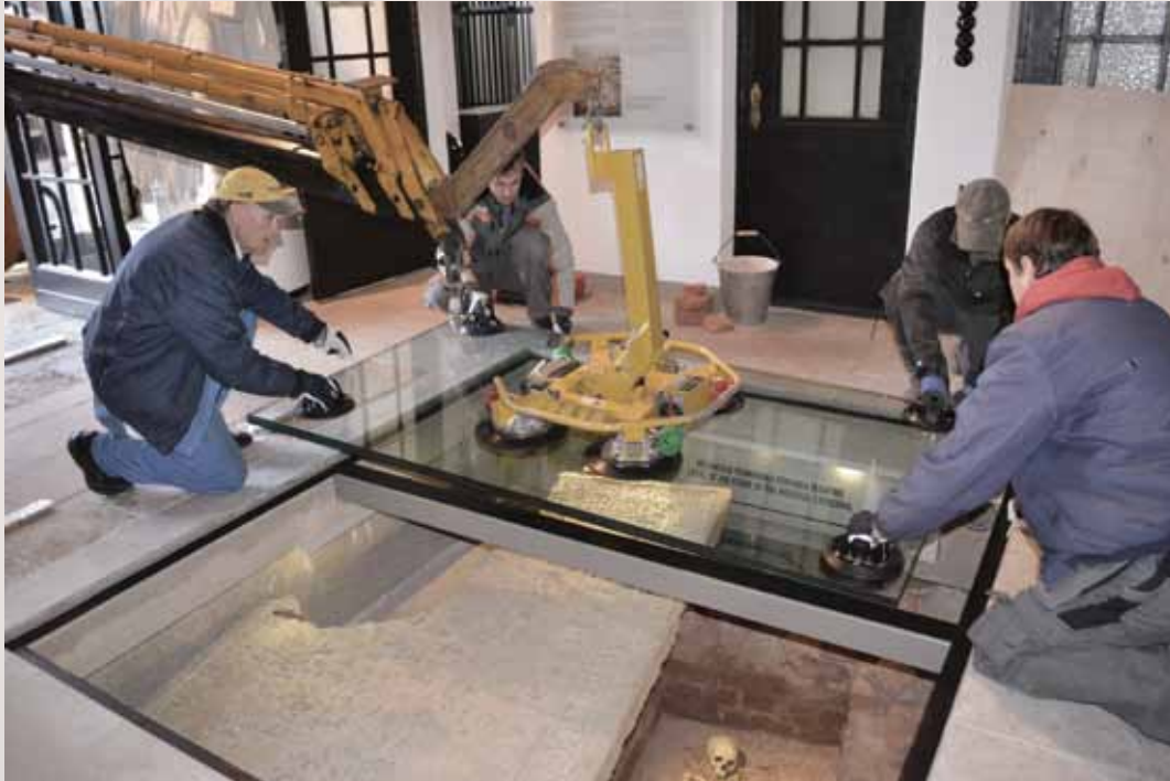
The pit dug in the Museum floor is overlaid by durable glass panes.
